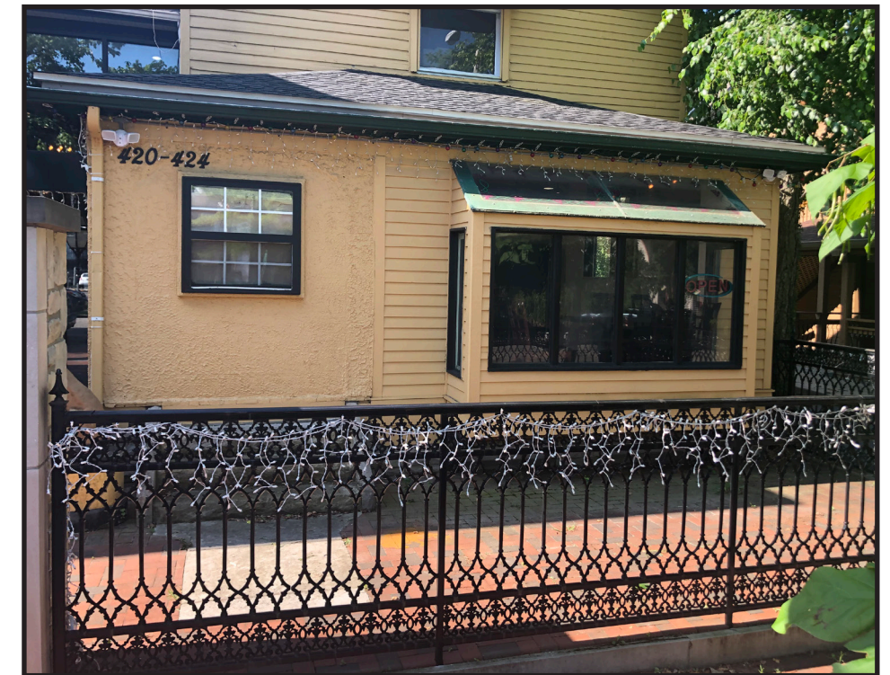
Incompatible: Enclosed Porch
