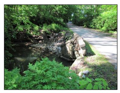
The existing bridge is relatively narrow and has concrete side rails with no approaching guardrail. The eastern concrete rail has broken and partially dropped out of position. It has been braced in place with metal brackets and supported by a crossing pipe. It has been in this condition for many years.
