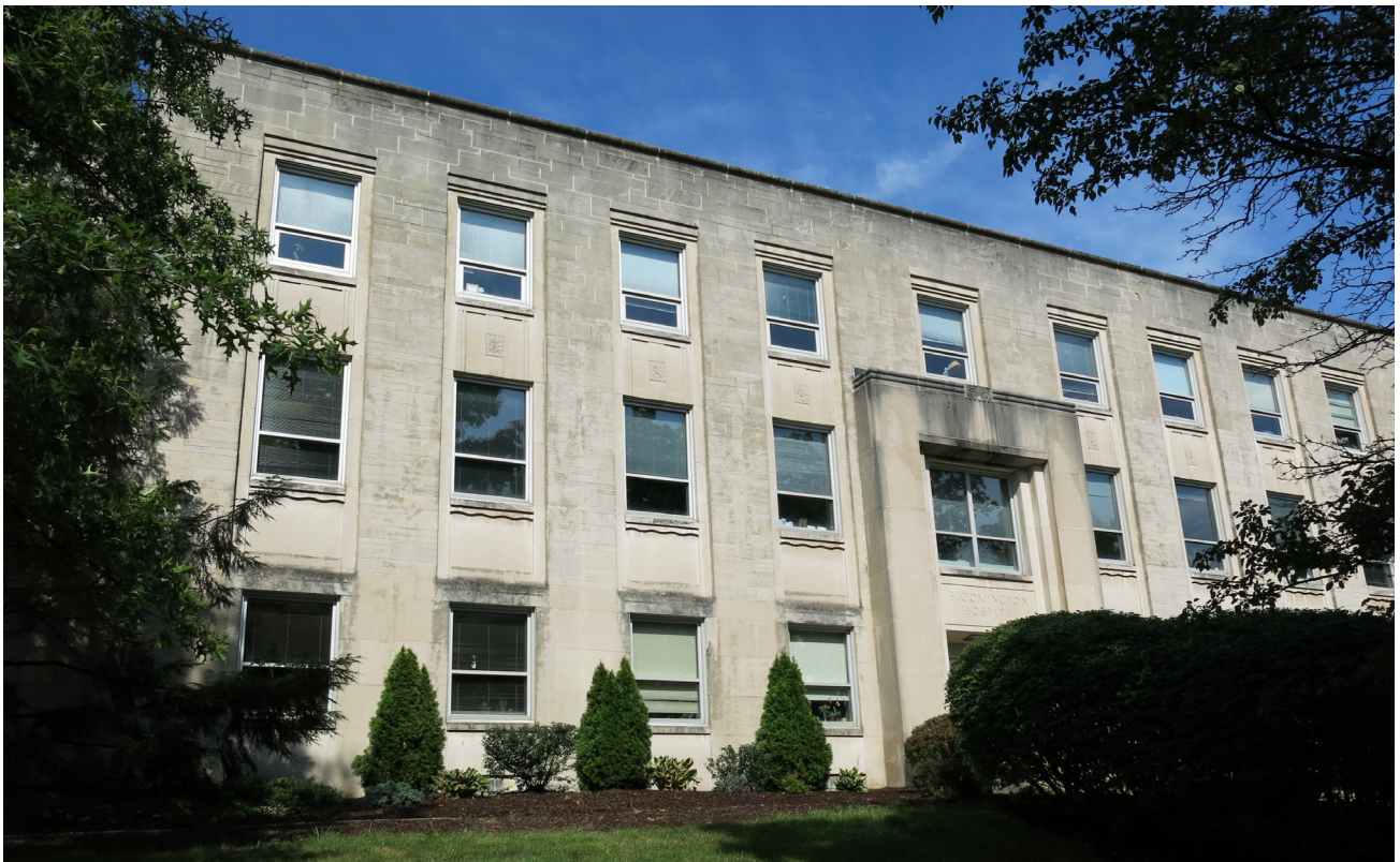
1947 wing, looking northwest, 2018
