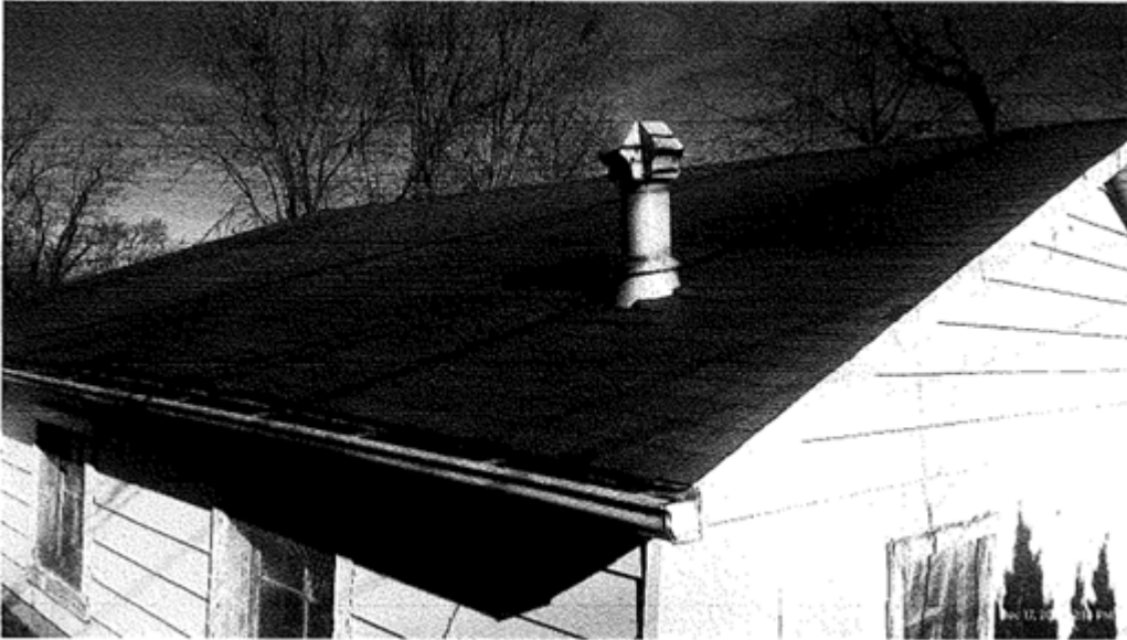
West half of roof looking northeast – Note humps and dips in roof framing
