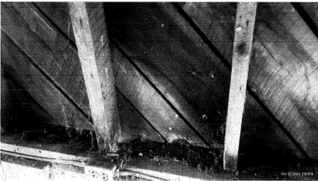
Damage at bottom wall plate
