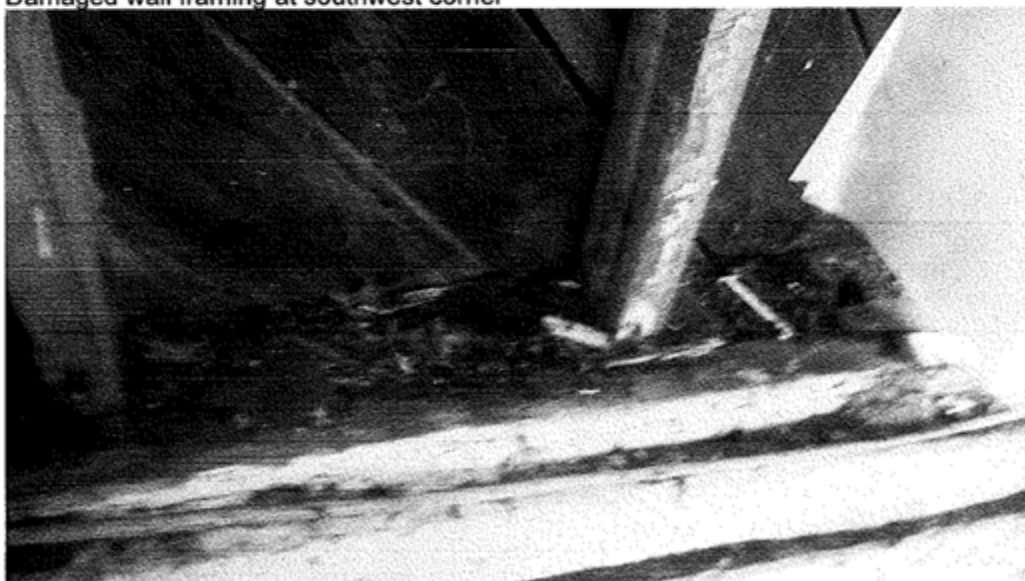
Termite damage at bottom of west wall
