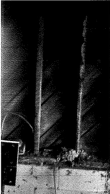
Termite damage wall framing
