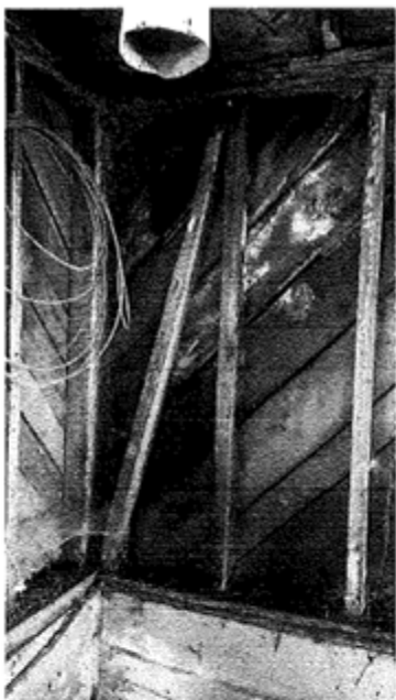
Damaged wall framing at southwest corner
