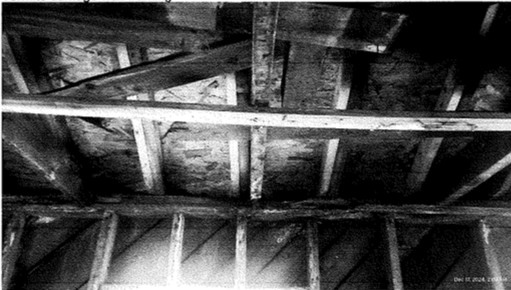
Water damaged wall framing on west wall
