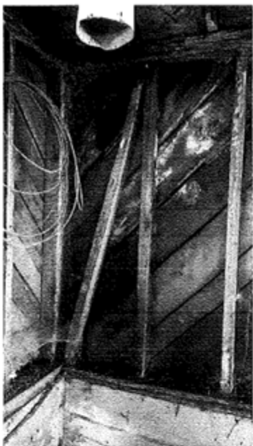
Damaged wall framing at southwest corner
