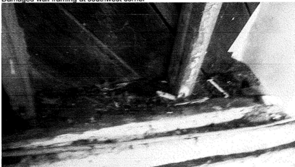
Termite damage at bottom of west wall
