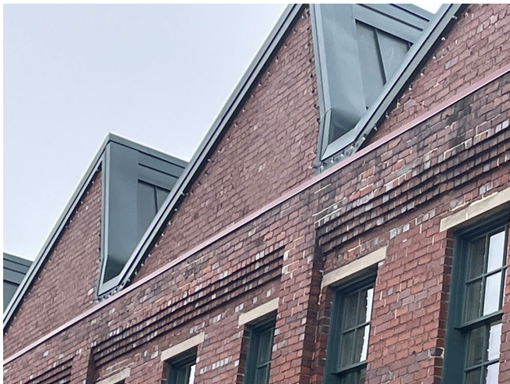
Corbel on City Hall with flashing
