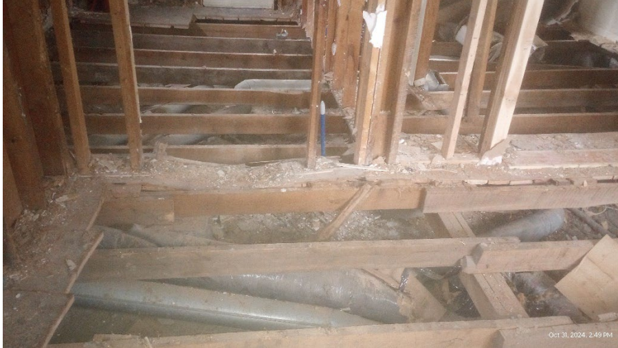
2 x 6 floor joists at 20 inch spacing in north unit – PHOTO (9)
