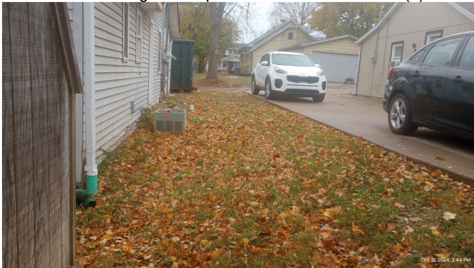
Grade sloping toward rear wall – PHOTO (4)
