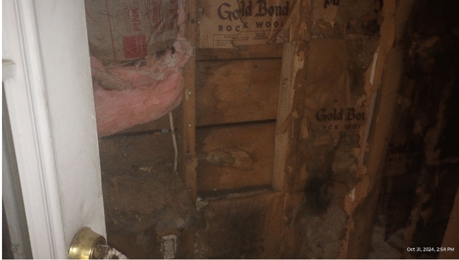
Wall sheathing and 2 x 4 studs – PHOTO (12)
