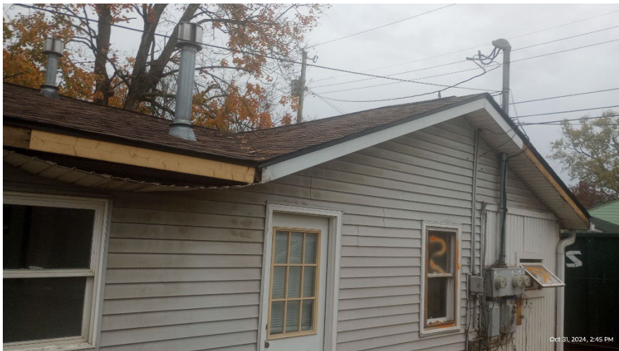
Soffit and fascia damage on east side- No roof gutter – PHOTO (6)
