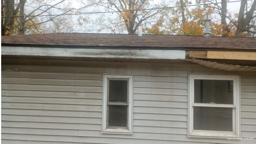
Damaged fascia and soffit on east wall – PHOTO (5)
