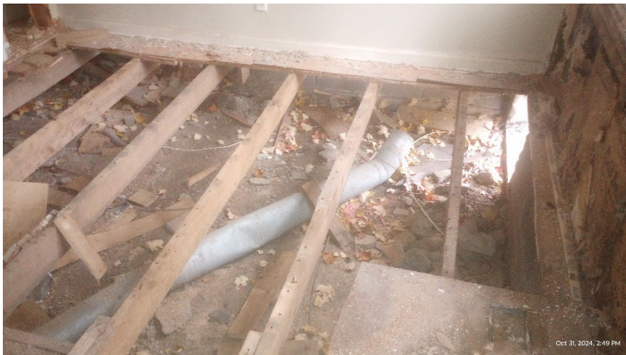
2 x 6 floor joists at 20 inch spacing along west side of north unit – PHOTO (10)
