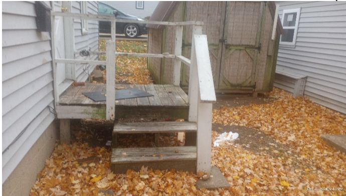
Deteriorated landing and steps on south side – PHOTO (3)
