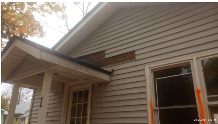
Missing vinyl siding on west side- "Insulbrick" siding below – PHOTO (1)
