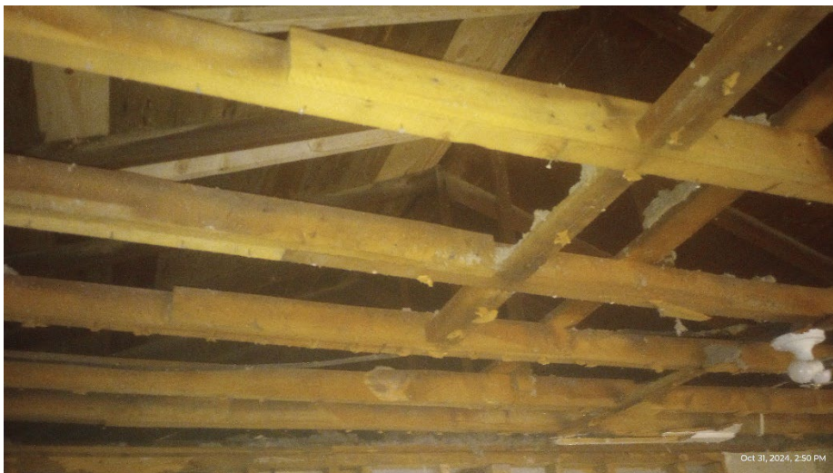
Spliced 2 x 4 ceiling joists over west living room in north unit – PHOTO (11)
