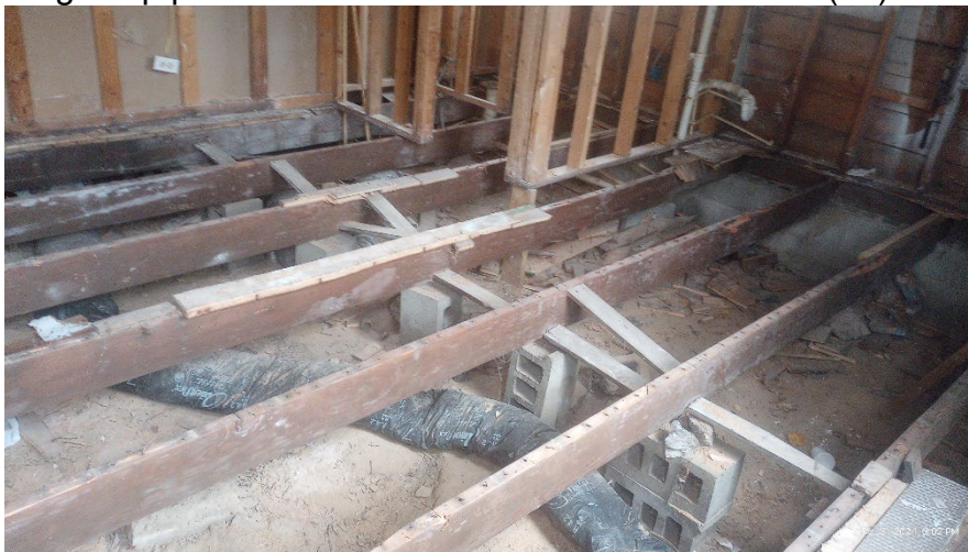
2 x 8 joists at 24 inch spacing in south unit looking east – PHOTO (14)
