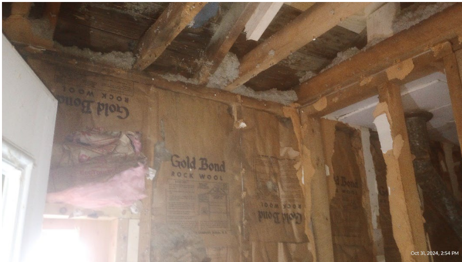
Single top plate for north wall in north unit – PHOTO (13)
