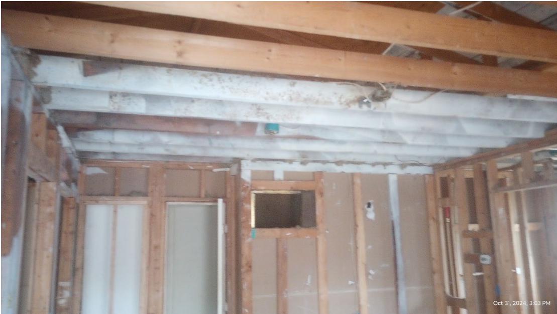
2 x 4 ceiling joists in south unit with 2 x 4 rafters above – PHOTO (16)
