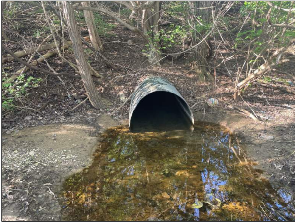
Photo 3: View looking south at the northern end (outlet) of the culvert.
