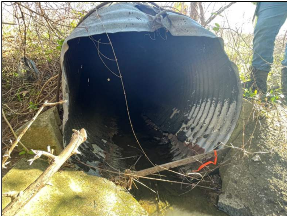
Photo 4: View looking north at the southern end (inlet) of the culvert.
