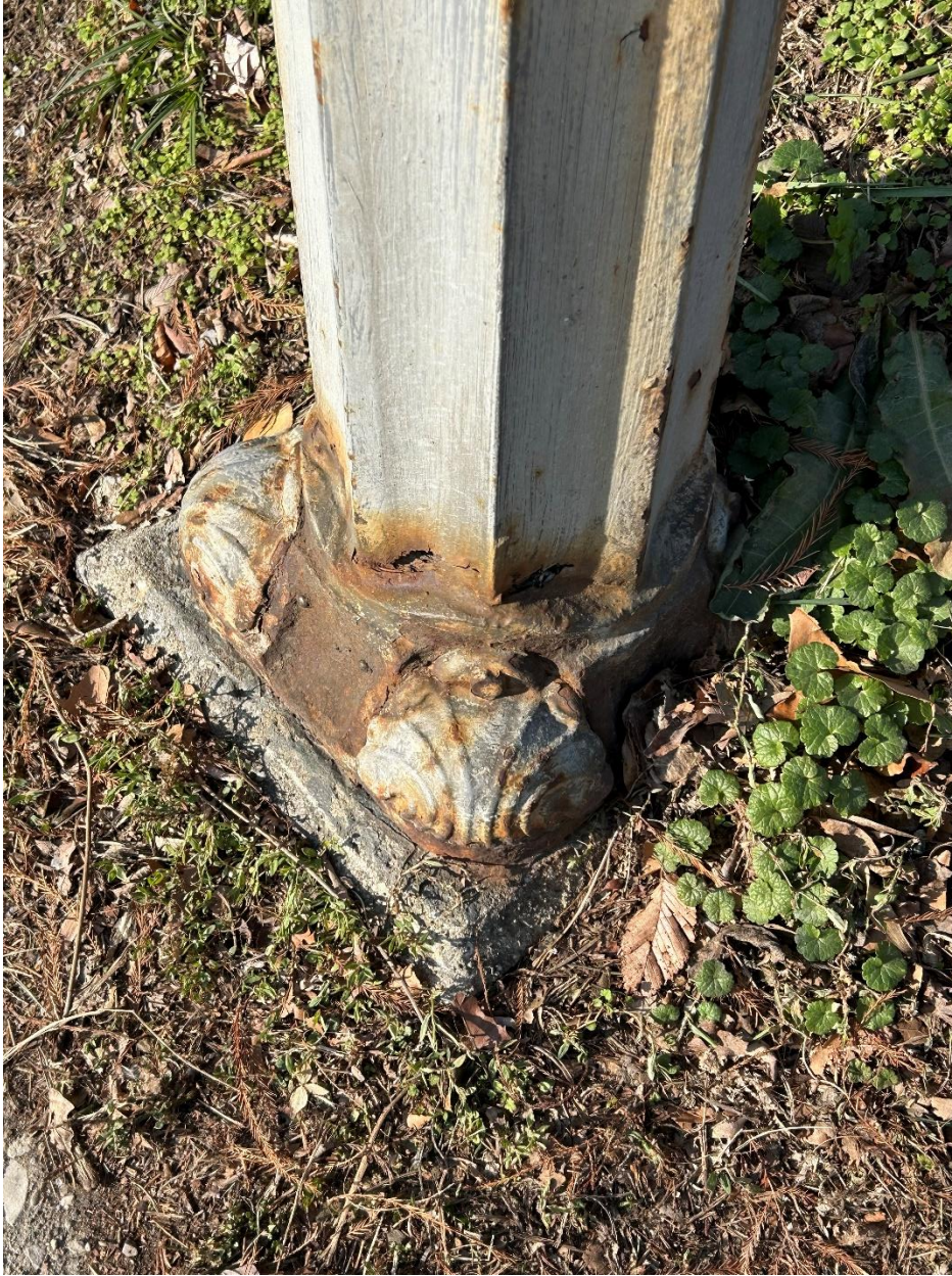
Base of street light showing decorative bolt covers
