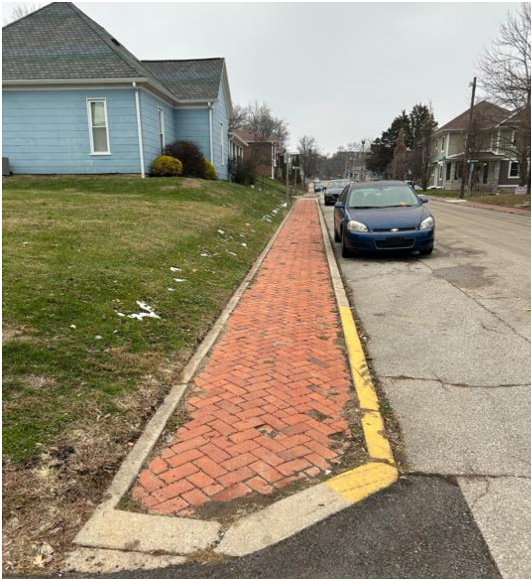
Brick Sidewalk Grant
