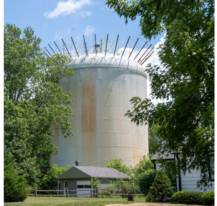
East Tank before recoating
