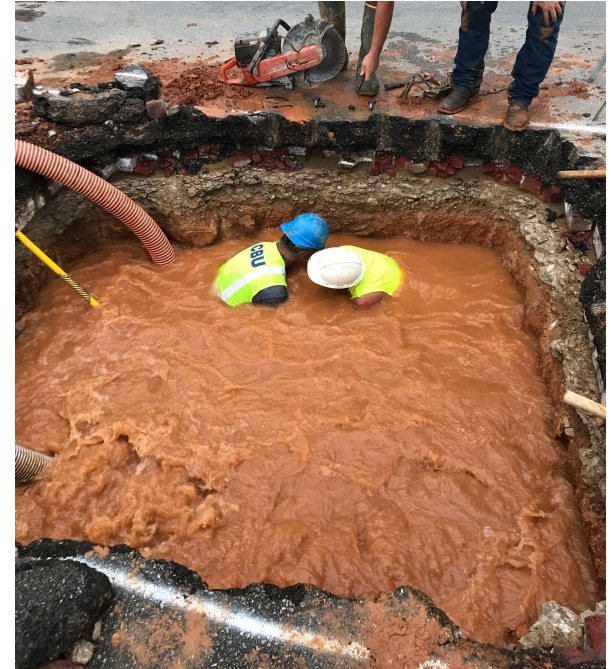
Utilities can be dangerous work
